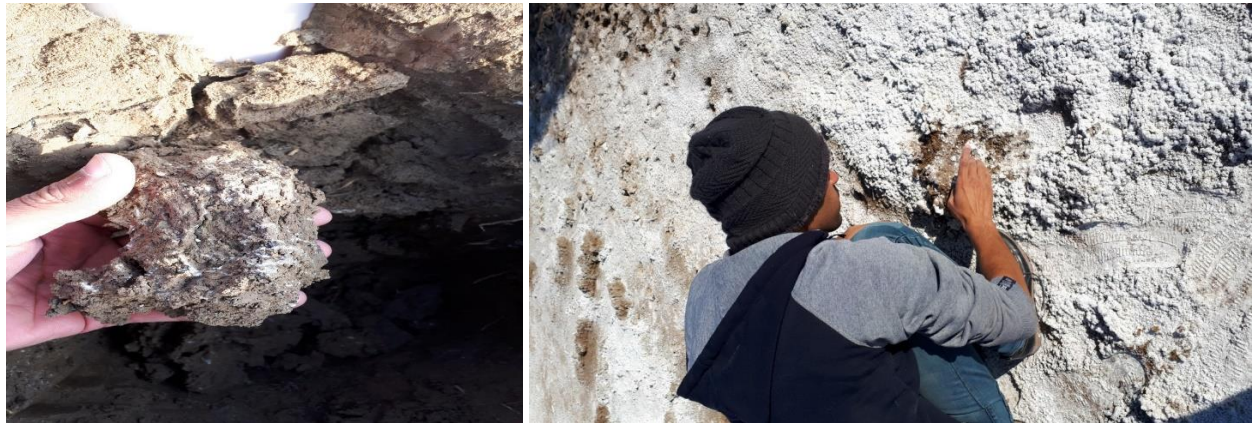
Fig 2: Inspection of salt-affected soil
